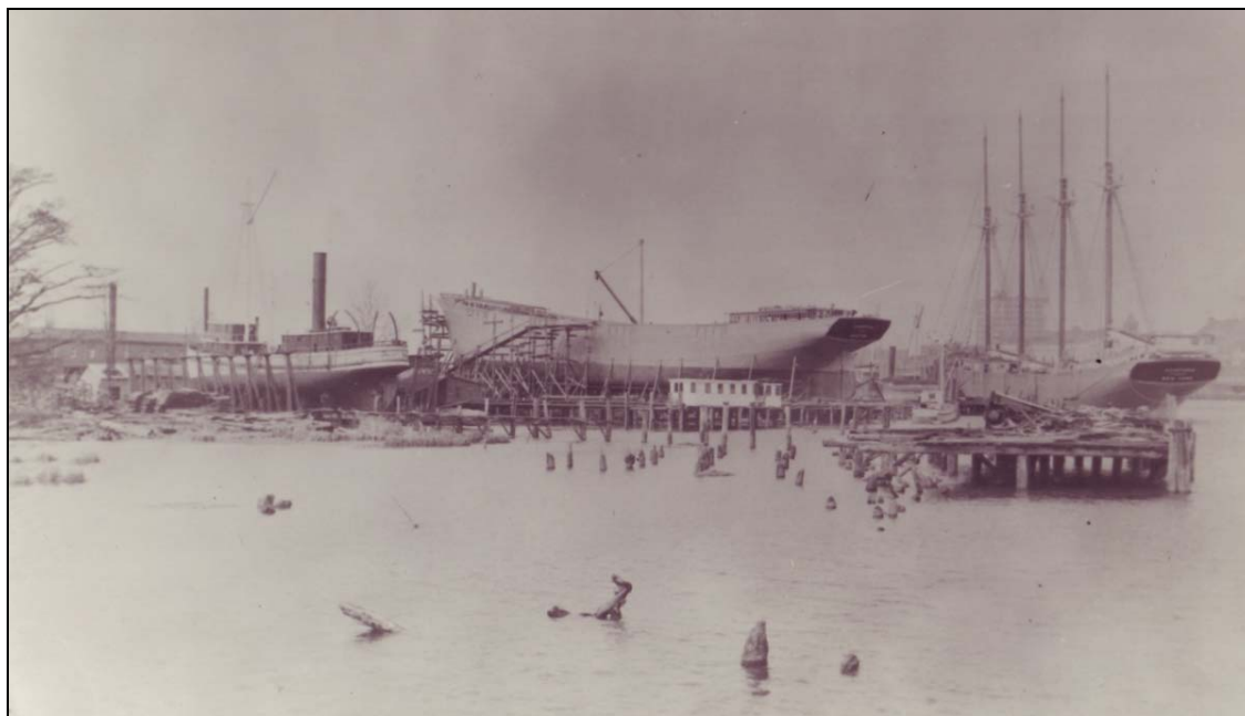
Figure 5.5: The Hoppauge and Commack under construction at the Wilmington Marine Railway on Eagles Island (Image courtesy of the North Carolina Underwater Archaeology Branch).
