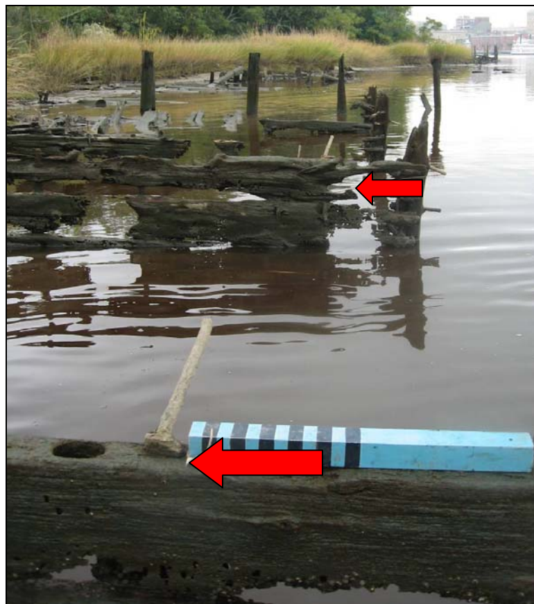
Figure 8.5: Evidence of crow bar utilization on wooden decking on Barge 2 (Image by Nathan Richards).
