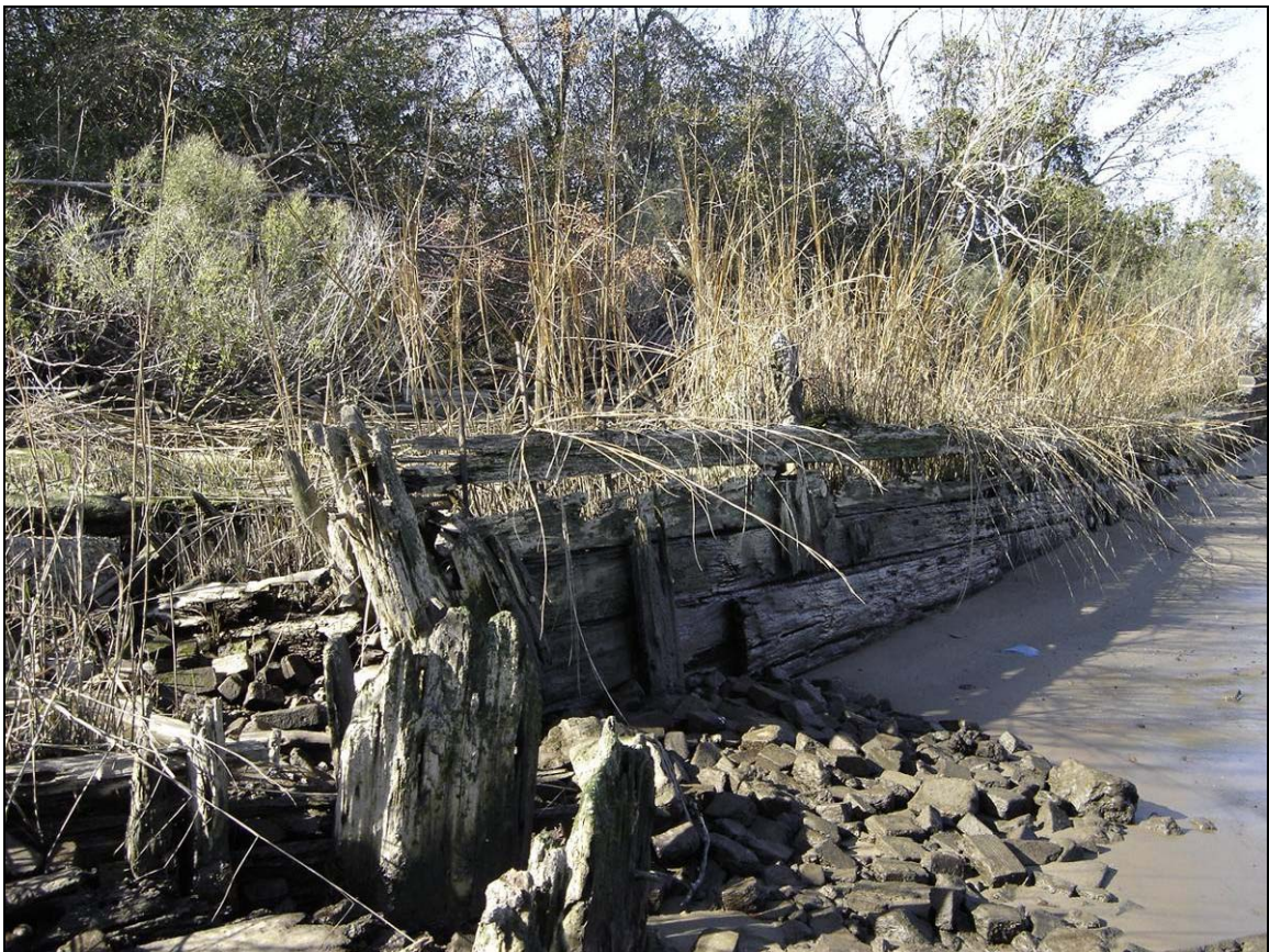
Figure 7.2: (Foreground) Bow of Bulkhead Tug, which is filled with brick and rock debris, abuts the Bulkhead Barge, creating a bulkhead for the railway to the north (Image by author).
