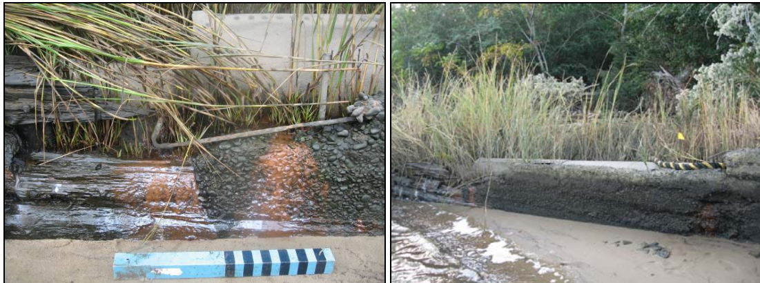
Figure 7.3: A concrete wall connects two barges, creating a bulkhead. (Left) The concrete wall built into the structure and fabric of the Bulkhead Barge and (Right) the concrete wall extending north out of the Bulkhead Barge towards Barge 3 (Images by author).
