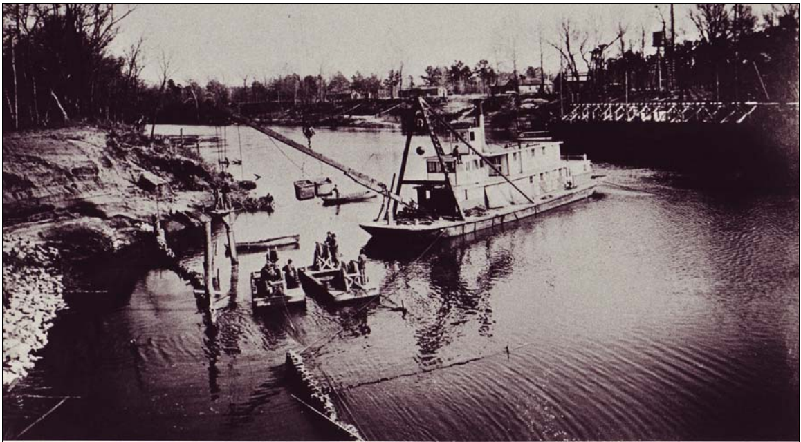
Figure 4.4: Corps of Engineers snag boat H.G. Wright making improvements on the Cape Fear River (Image courtesy of the North Carolina Underwater Archaeology Branch).
